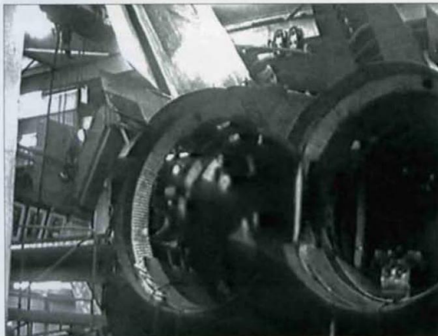
These pictures show one of the Ye-155 prototypes (not the first one, as indicated by the raked fin tips) taking shape at the Mikoyan OKB's experimental plant. Note how the circumferences of the engine bays intersect in the nozzle area. The lower right picture shows the internal structure of one of the fuselage fuel tanks.
